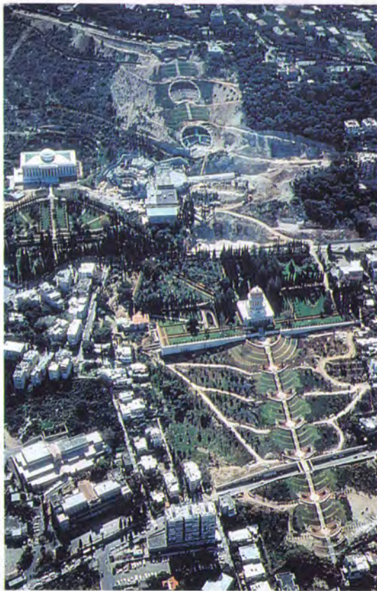
Aerial photograph showing dramatic progress on the Arc and Terraces Projects, March 1996.
