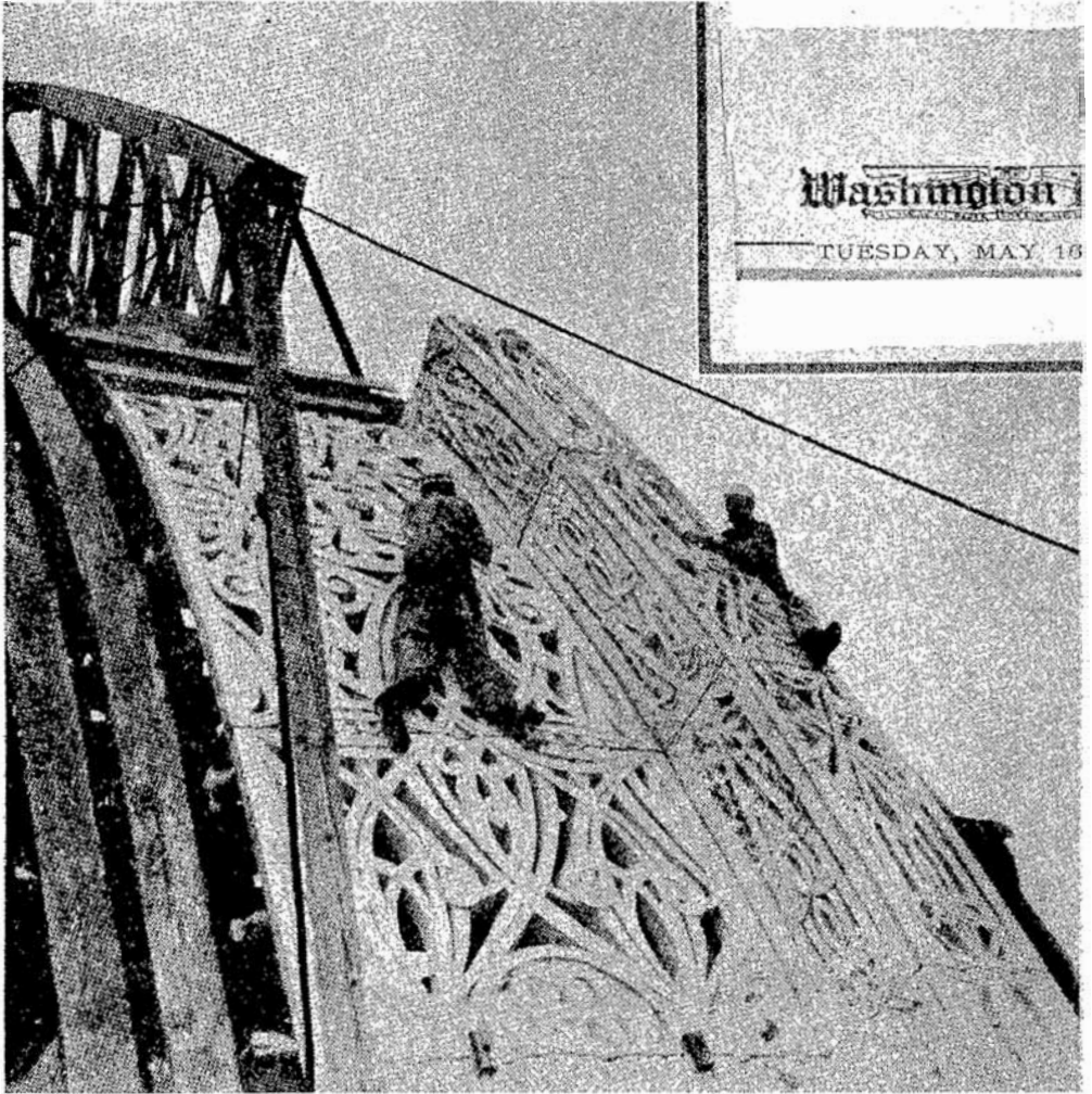
Work on Exhibit—Workmen fit together plaster sections of the full-size model of the dome for the Bah'i Temple of Light.
