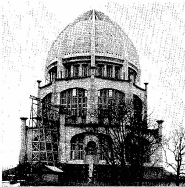
Figure 27.—The dome as now assembled—the remainder of the structure still to be completed.
