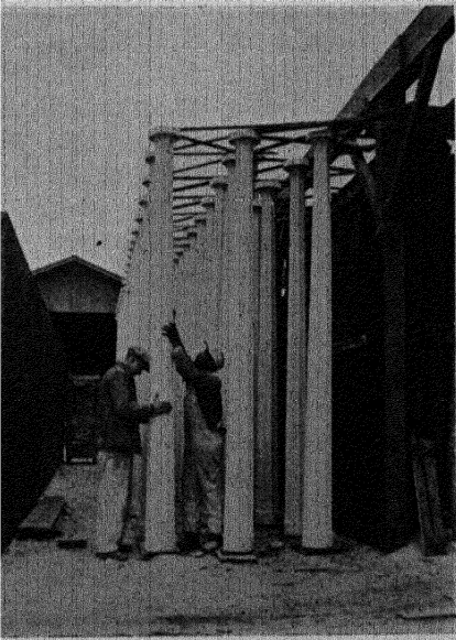
Finished Units for Gallery Section.
