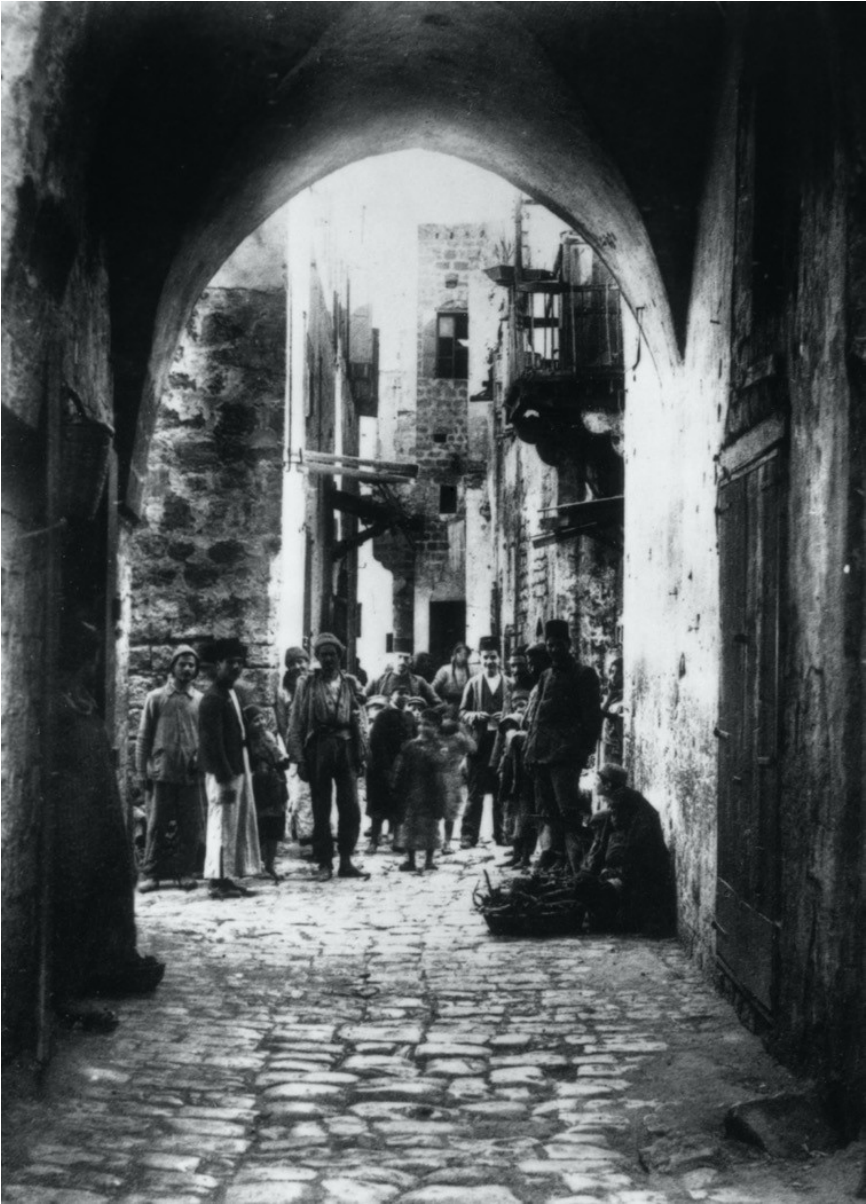
Figure 16: A street of 'Akká at the beginning of the 19th Century. Courtesy: Bahá'í World Centre.
