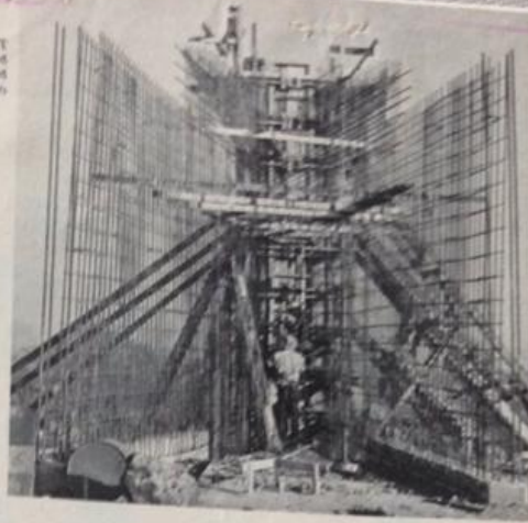
All openings were left ungrouted for free air flow. This formwork was shotcrete to form a shell over the opening in the apex of the dome.
