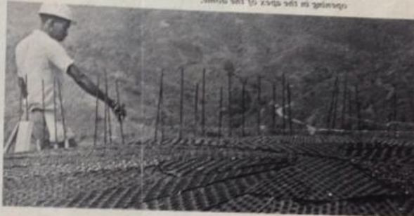
All openings were left ungrouted for free air flow. This formwork was shotcrete to form a shell over the opening in the apex of the dome.
