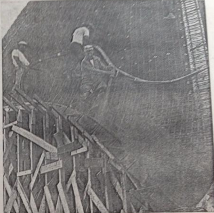
Early stages in the gunite process on the dome.
