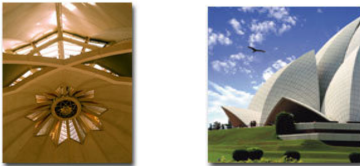
Figure 3.75: (l-r) Opening on top of the Dome with exhaust fans to aid natural ventilation through horizontal openings (r) at the basement level
