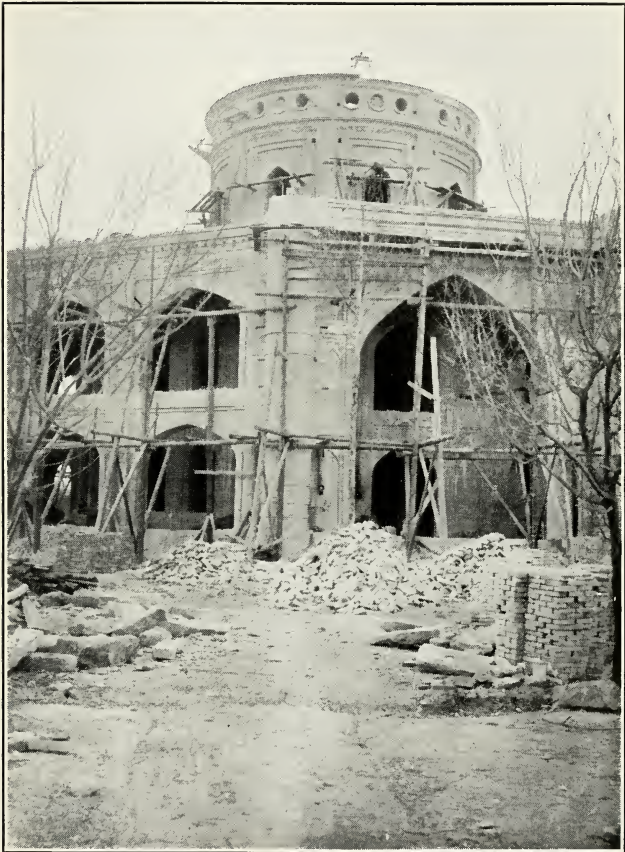
THE MASHRAK-EL-AZCAR OF ESHKHABAD UNDER CONSTRUCTION.
