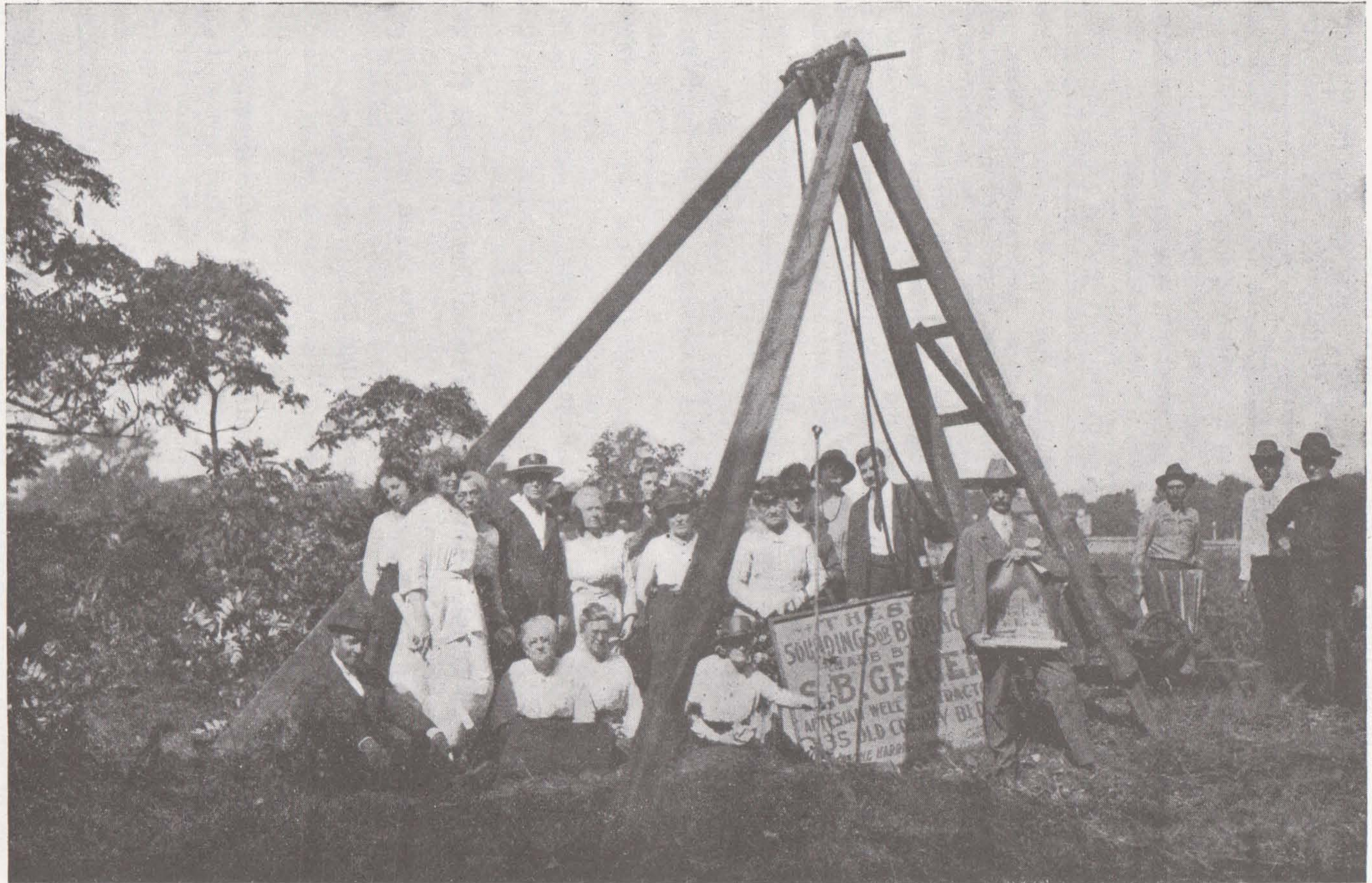
BAHAI FRIENDS AND WORKMEN ON MASHREKOL-AZKAR GROUNDS WHEN BORING COMMENCED, SEPTEMBER 24, 1920.
