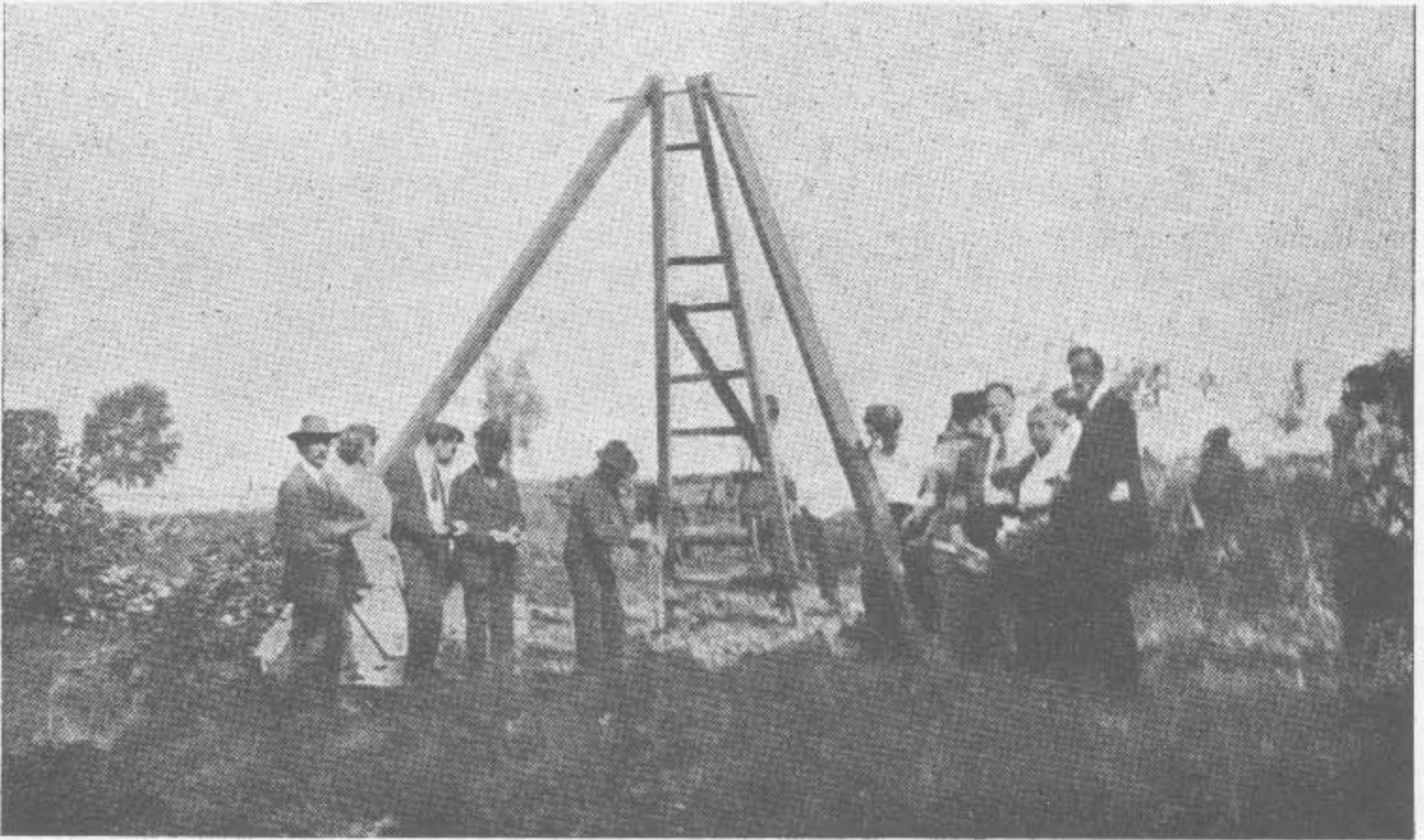
BEGINNING FIRST BORING—FRIENDS HOLDING SOIL IN HANDS
