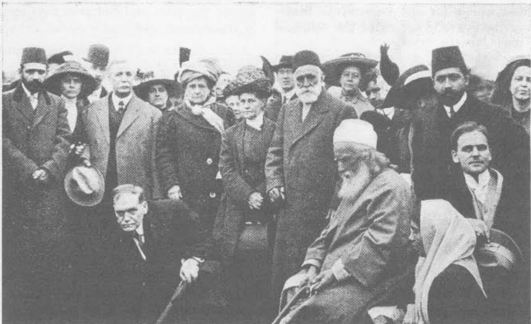
Breaking the ground—each race and nation in turn taking hold of axe and shovel.
