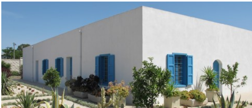
Exterior view. The two windows seen on each side of the corner wall, are the windows of the room Bahá'u'lláh used to occupy when in the Junaynih Garden.
