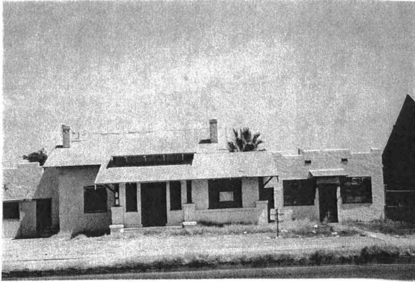
The former Bugbee home and its Assembly Hall addition as it appeared in 1989, abandoned and deteriorating.
